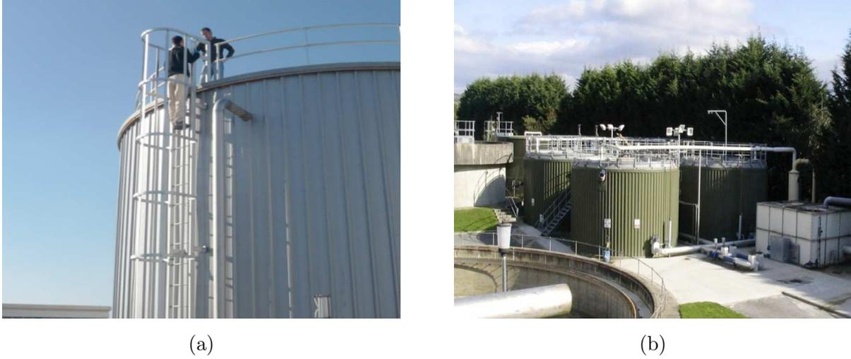
**Figure 3:** (a) *Stand-alone reactor plant;* (b) *Two reactor in series design.* The two designs displayed correspond to plants located in Tudela (Navarra, Spain) and Killarney (Co. Kerry, Ireland), respectively.
